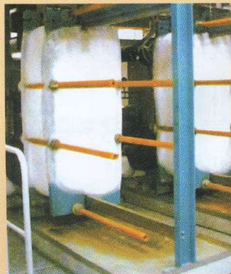
Figure 9: In case of freezing of a PHE, plates and gaskets do not get damaged.
